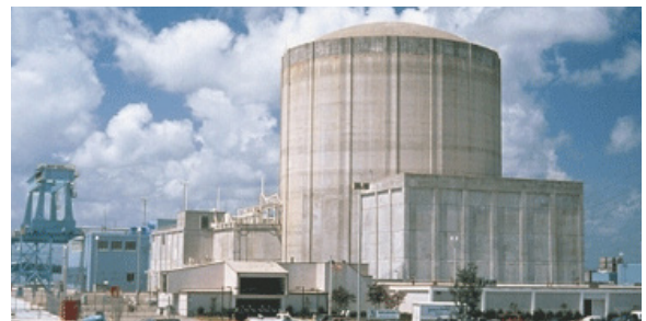
WATERFORD 3 NUCLEAR POWER PLANT, LA
