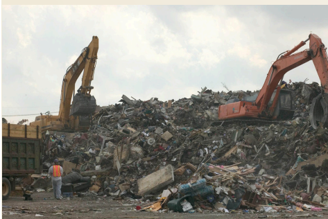
DEBRIS STAGING AREA, NEW ORLEANS
