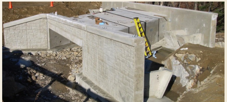
AFTER MITIGATION: NEW CULVERT WITH PROTECTIVE HEADWALL
