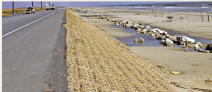
AFTER MITIGATION: ROAD NEAR HOLLY BEACH EROSION CONTROL MATS
