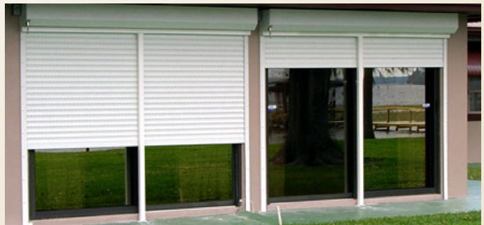
AFTER MITIGATION: ROLL-DOWN SHUTTERS ADDED TO STOREFRONT
