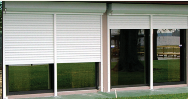
AFTER MITIGATION: ROLL-DOWN SHUTTERS ADDED TO STOREFRONT
