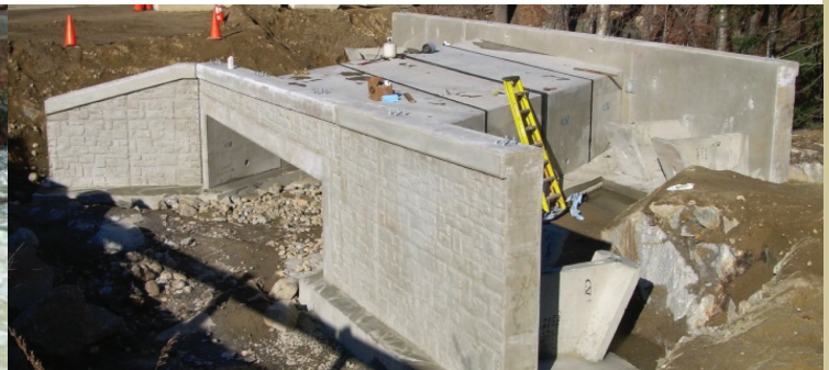
AFTER MITIGATION: NEW CULVERT WITH PROTECTIVE HEADWALL
