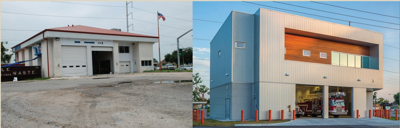
ST. BERNARD IMPROVED PROJECT – CHANGING A ONE-STORY FIRE STATION TO A TWO-STORY FIRE STATION
