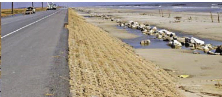
AFTER MITIGATION: ROAD NEAR HOLLY BEACH EROSION CONTROL MATS
