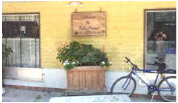
Figure 20 - This home in Jefferson Parish, LA has permanent shields sealing the space under the windows.
