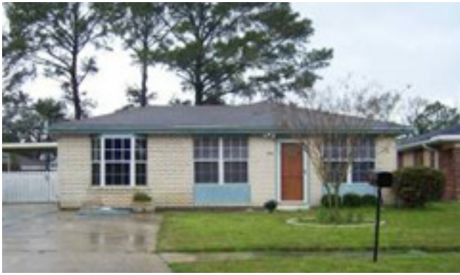
Figure 19 - This dry floodproofed building in Mandeville, LA has the walls waterproofed and removable shields placed in front of the windows.
