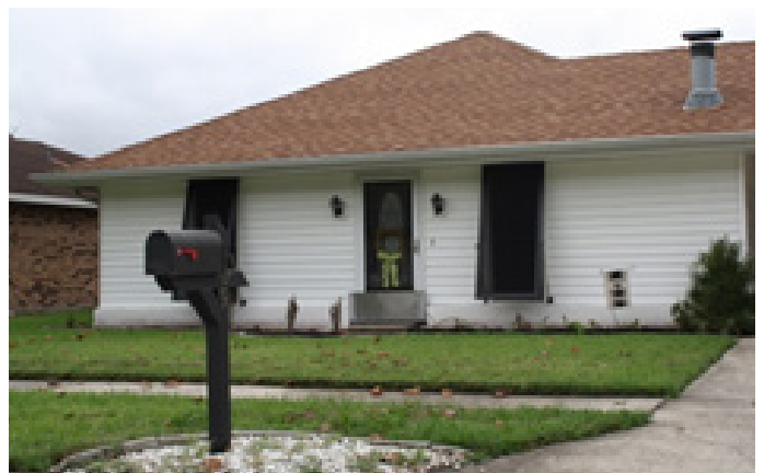
Figure 18 - This Terrebonne Parish home has a steel door to keep flood waters out.
