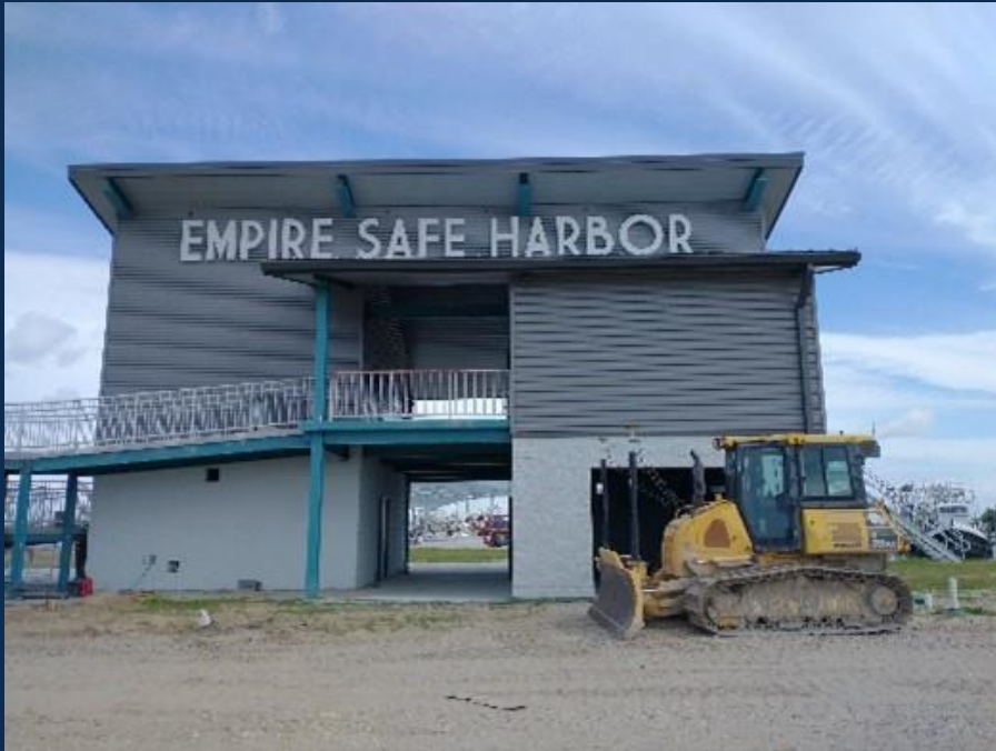
Figure 5 -Harbor of Refuge Design & Construction — Infinity Engineering Consultants, LLC. ( infinityec.com )
