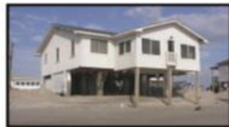
Figure 17-2. This coastal building suffered extensive damage to the enclosed lower area.
